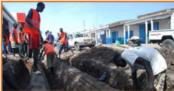
Constructing a new drainage system in Sudan.
