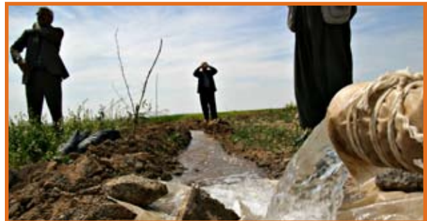
A reconstructed irrigation system in Iraq.
