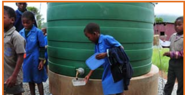
Using a new water storage system in Swaziland.
