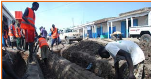
Constructing a new drainage system in Sudan.
