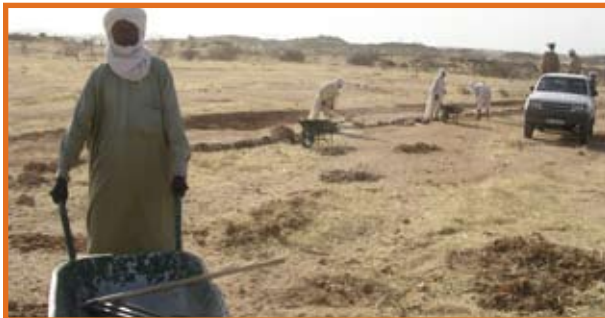
Rehabilitating a road in Chad.
