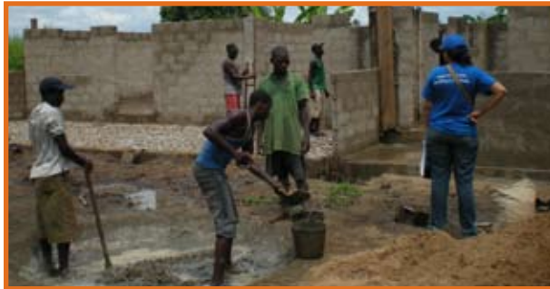
Building a school in Mozambique.
