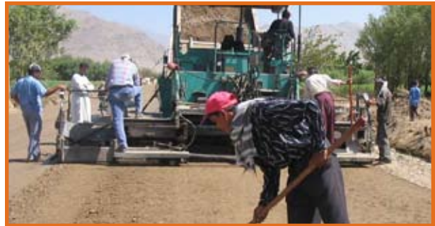
Reconstructing a road in Afghanistan.
