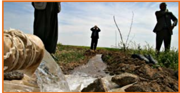
A reconstructed irrigation system in Iraq.
