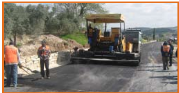
Road construction on the West Bank.
