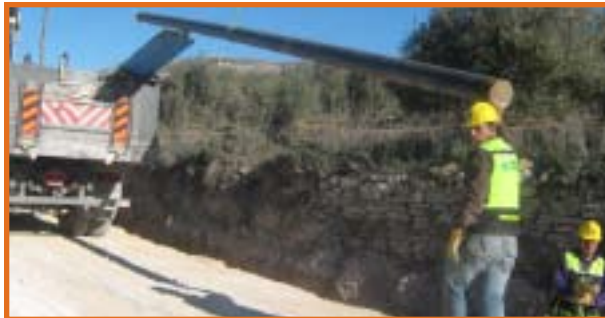
Laying pipes for a water project in the West Bank.
