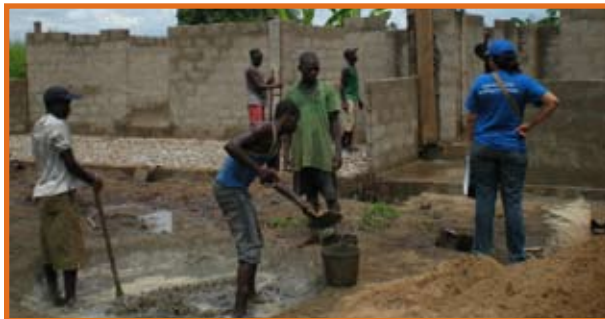
Building a school in Mozambique.
