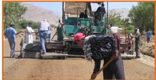
Constructing a road in Afghanistan.
