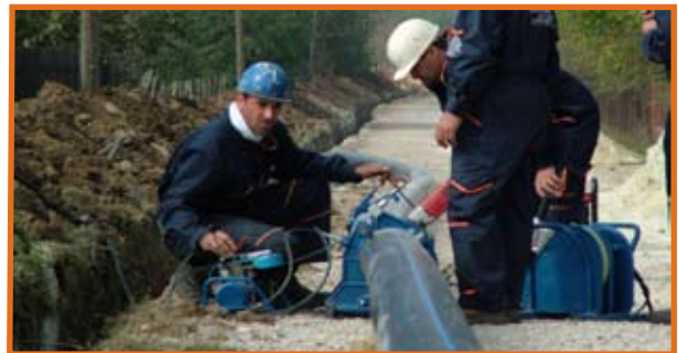
Rebuilding the infrastructure in Serbia.
