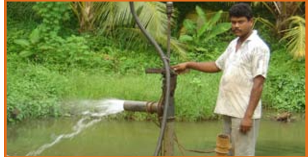
Installing a water system in Sri Lanka.
