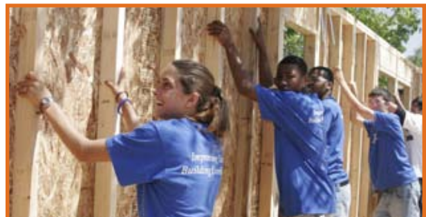
At-risk youth build a home in Mississippi.
