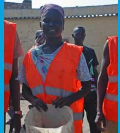
A woman working on the drains construction project in Malakal.
